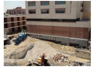
of the debris. The West building has been demolished to the first floor level. When the utilities now running through the West building to the North building have been re-routed, the West building will continue demolition to the basement floor. When that's completed, crews will punch holes in the concrete flooring to allow water drainage, but the basement floors will not be taken out. After that, the next step is to backfill the large holes where both building once stood.
